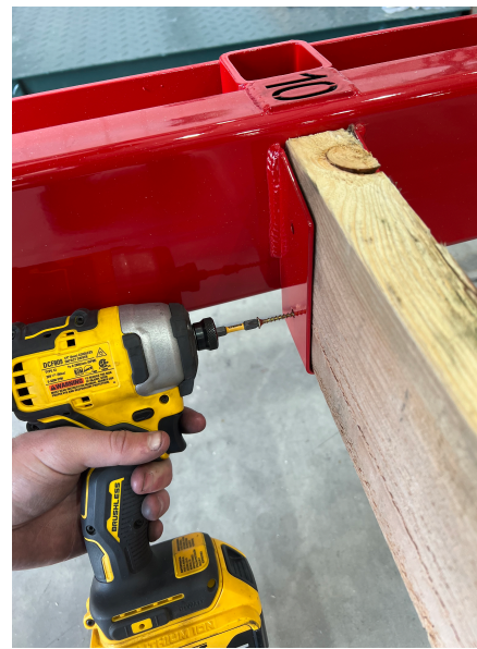
Place One Screw 1 1/4" Long Into Each Rafter and Hanger
